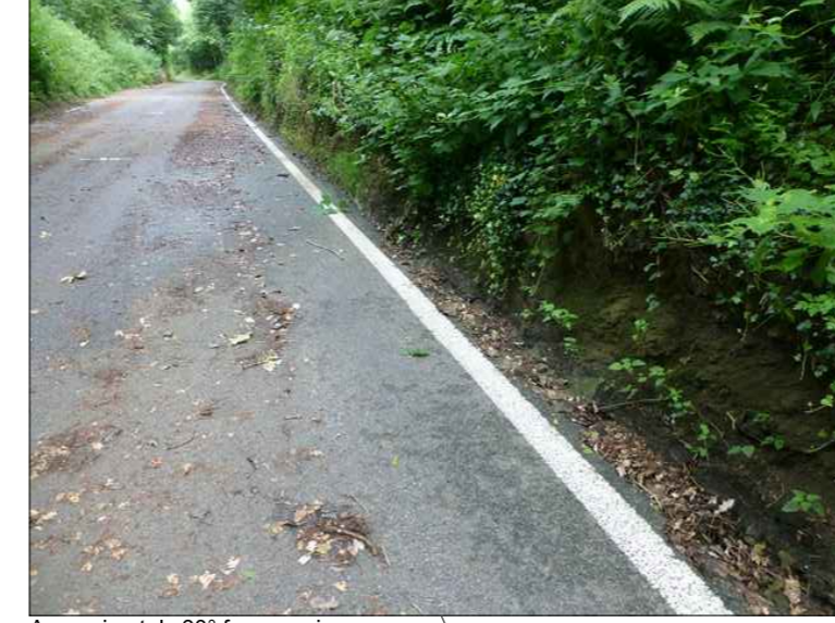
Approximately 50° face varying in height from 0.5-2m high at the toe of the slope
