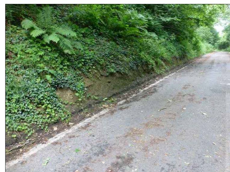
Approximately 75° face 0.7m high at the toe of the slope
