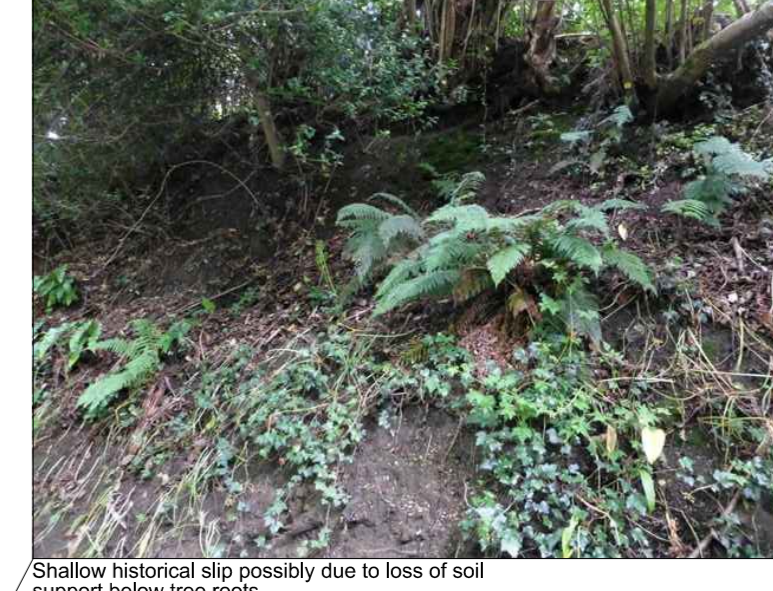
Shallow historical slip possibly due to loss of soil support below the road
