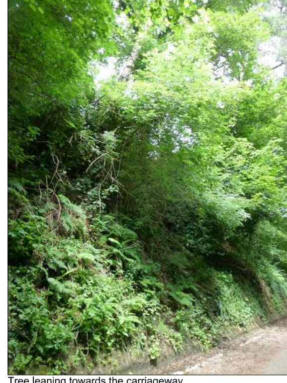
Tree leaning towards the carriageway
