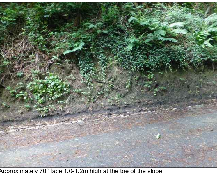
Approximately 70° face 1.0-1.2m high at the toe of the slope
