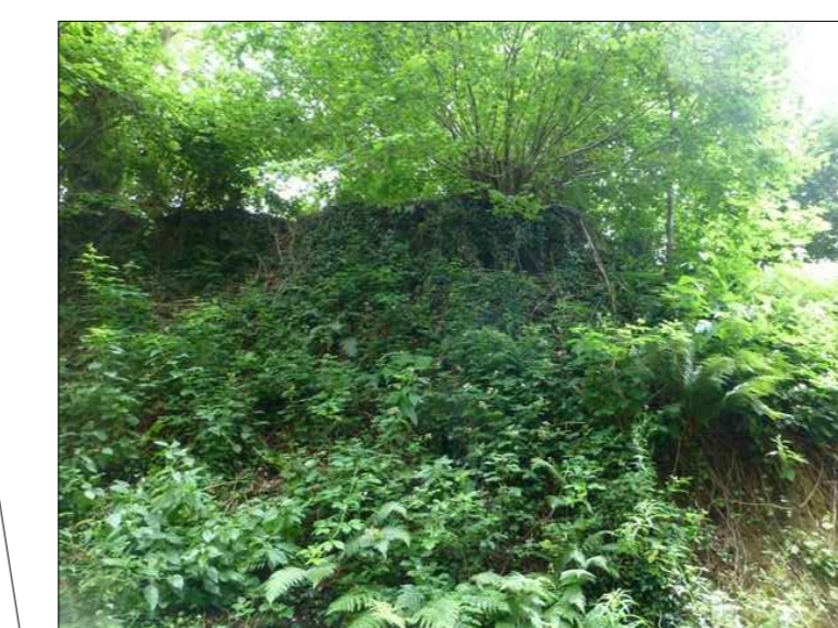
Overhanging tree at crest of slope
