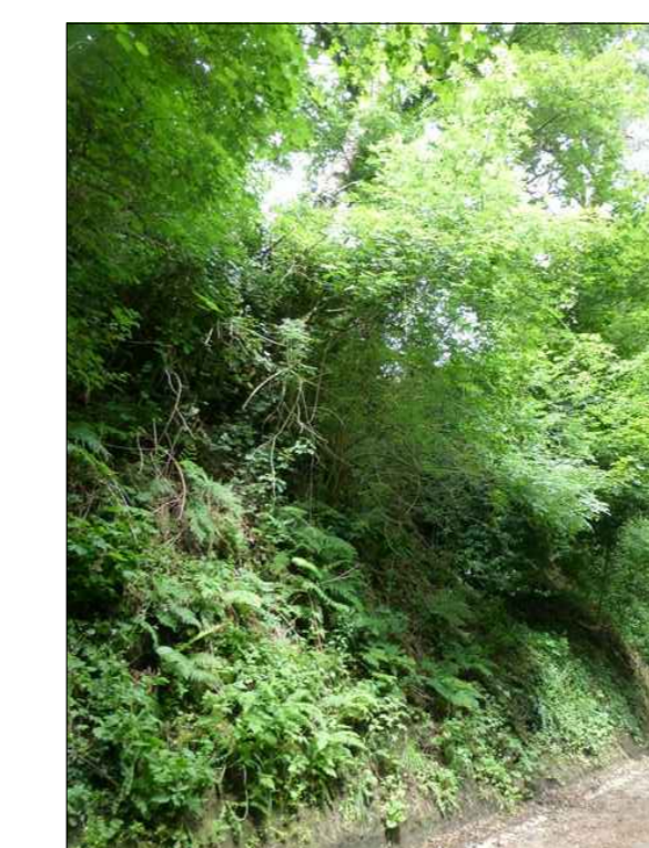
Trees leaning towards the carriageway
