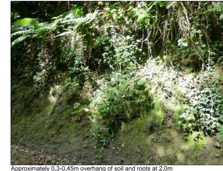
Approximately 1.3-1.6m overhang of soil and roots at 2.0m above the carriageway
