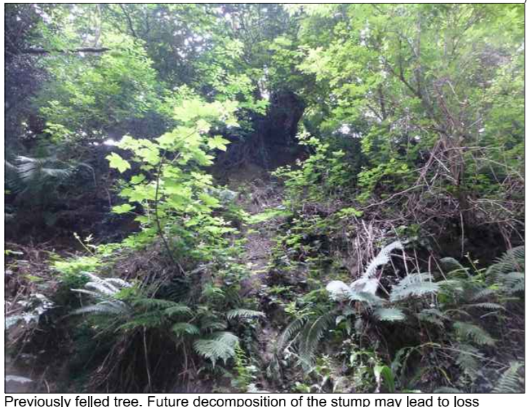
Previously felled tree. Future decomposition of the stump may lead to loss of soil support and subsequent slope failure
