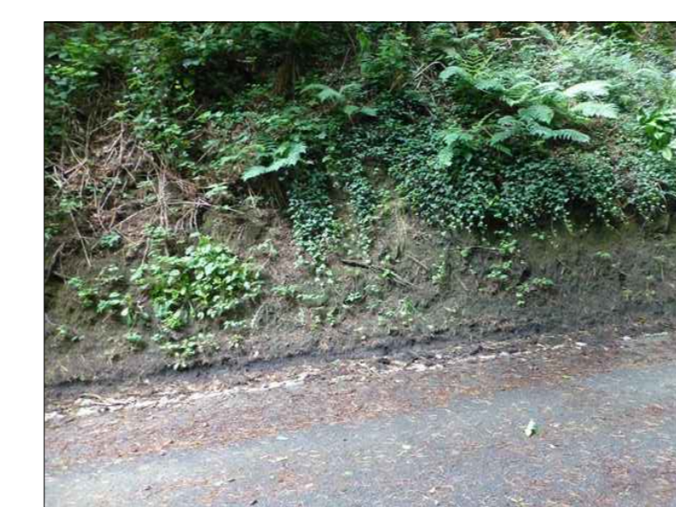
Approximately 70° face 1.0-1.2m high at the toe of the slope
