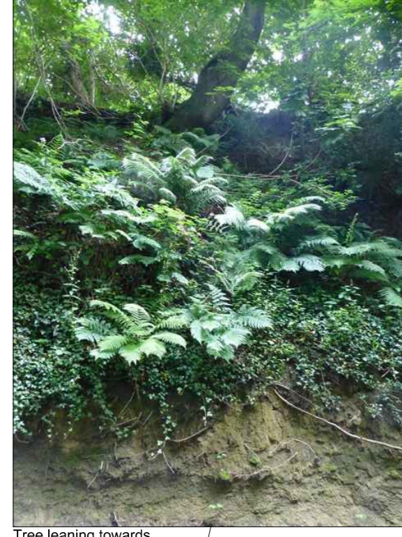
Tree leaning towards the carriageway
